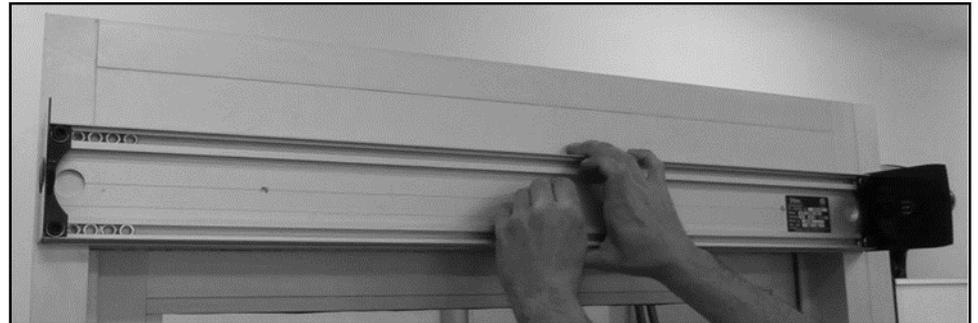
Step 3) Drill center mount hole to hang back plate
